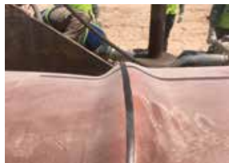
FIGURE 3. After wrinkling a pipe coated with Pipeclad 2060 MRO ARO, inspectors found the coating to be fully intact.
