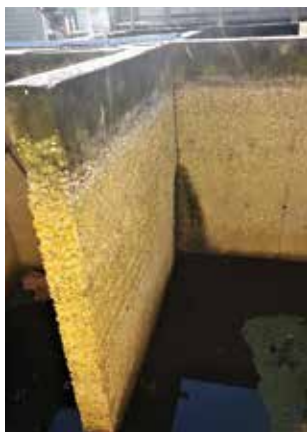
Corrosive contents can wreak havoc on concrete assets like this chlorine contact chamber in which the basin and baffles were severely deteriorated—almost to the point of crumbling (left). Following surface preparation, applicators added mortar to restore the concrete to its original plane before applying an elastomeric polyurethane liner with no seams, voids or pinholes (right).
