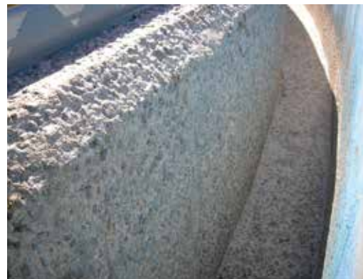
Lining a concrete clarifier with either a rigid epoxy or elastomeric urethane (left) will prevent the severe deterioration that an unlined concrete clarifier will experience (right).
