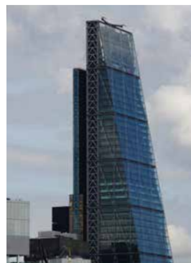
In fireproofing the structurally complex Leadenhall Building in London, applicators coated the steel in the shop rather than in the field.
