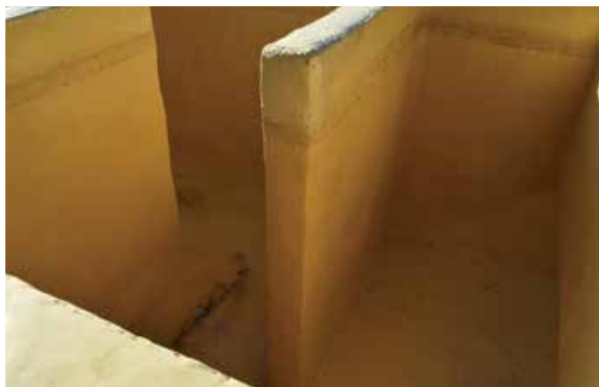
Corrosive contents can wreak havoc on concrete assets like this chlorine contact chamber in which the basin and baffles were severely deteriorated—almost to the point of crumbling (left). Following surface preparation, applicators added mortar to restore the concrete to its original plane before applying an elastomeric polyurethane liner with no seams, voids or pinholes (right).
